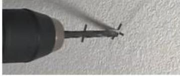
2. Remove the debris and clean the holes using the dust pump.
